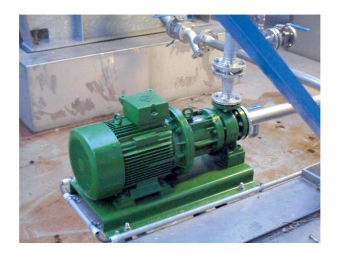
Sealless Magnetic Coupled Centrifugal Pumps acc. to EN 22858 / ISO 2858
